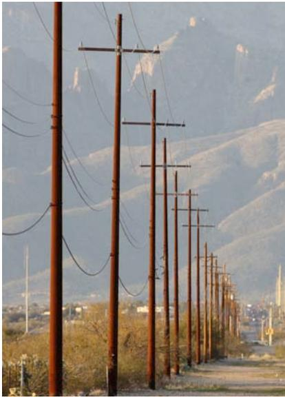
Since moving to steel poles almost exclusively, TEP has noted improvement of system reliability. Wind is the most severe natural power system problem on our system.
